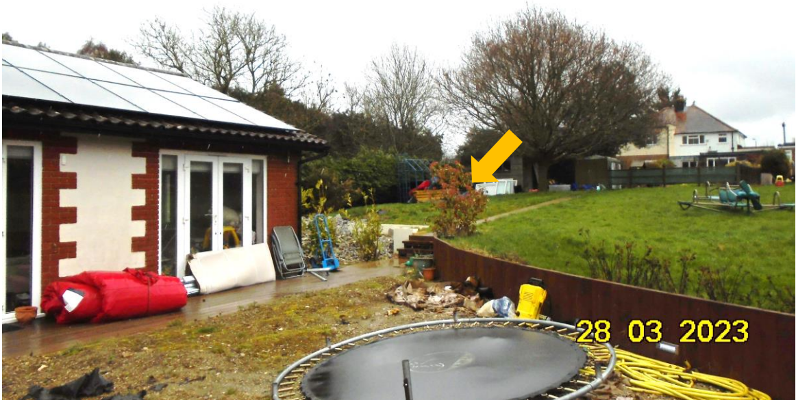
Photo 2: Existing garden (viewed from the garage).
