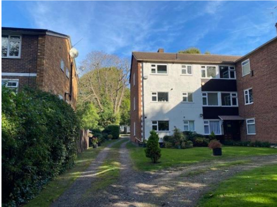
Figure 15 – host building on left and No. 47 on right
