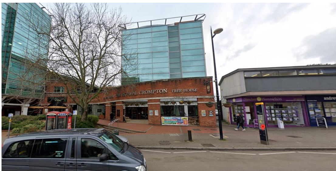
Figure 3 – front of building
