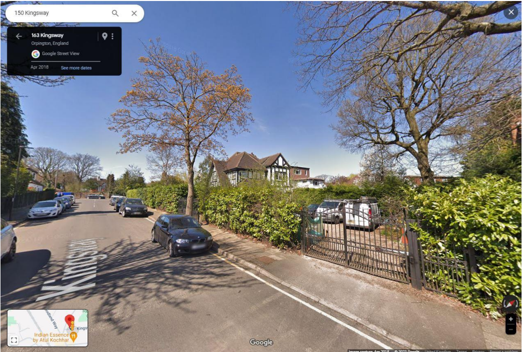
Photograph 1. Previous 150 Kingsway boundary (circa April 2018).
